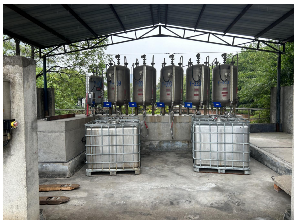
甲类罐区分装棚
